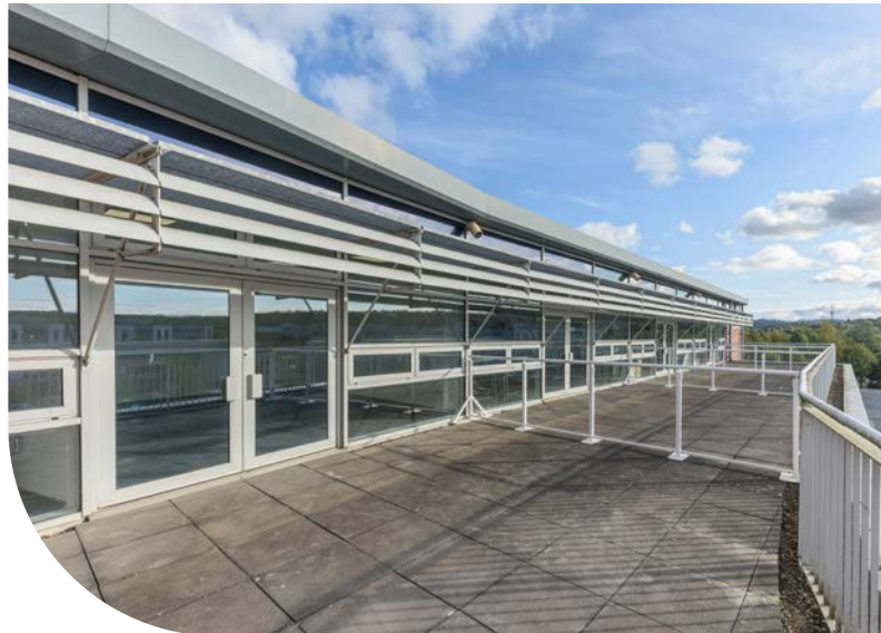
Suite 3 second floor terrace with allocated outdoor space
